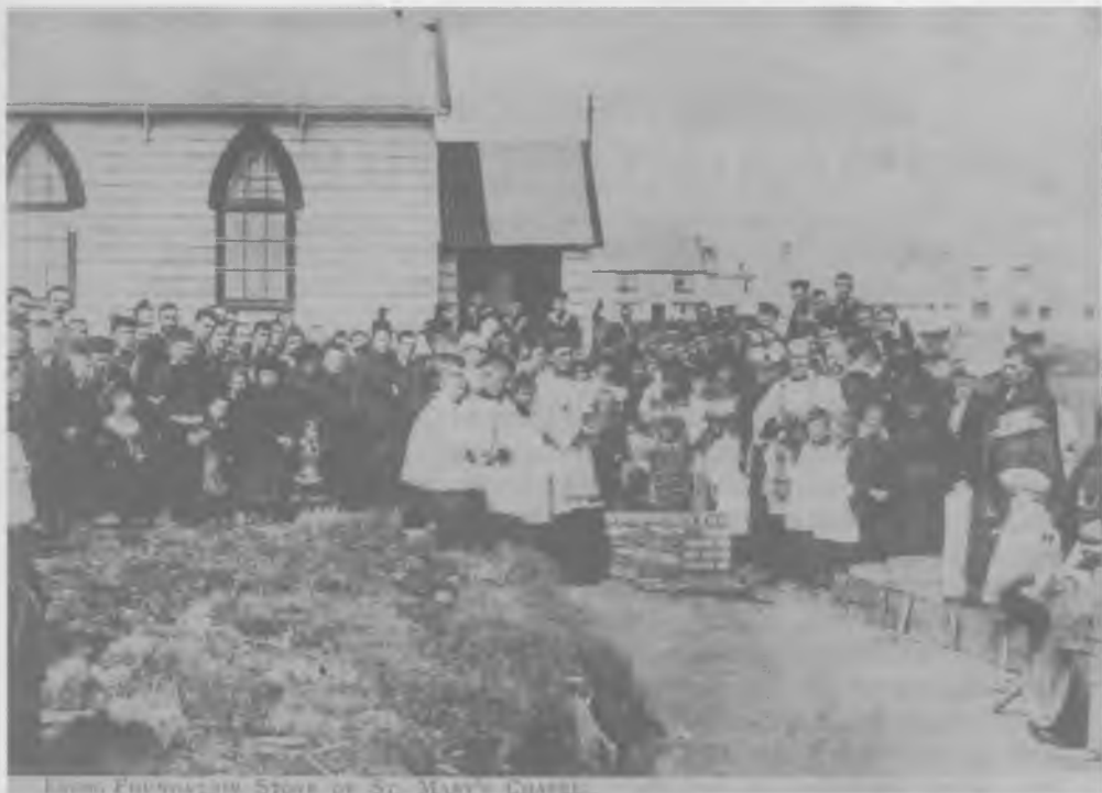
Laying Foundation Stone of St. Mary's Church. Laying the Foundation Stone of the present St Mary's Church, 1899
